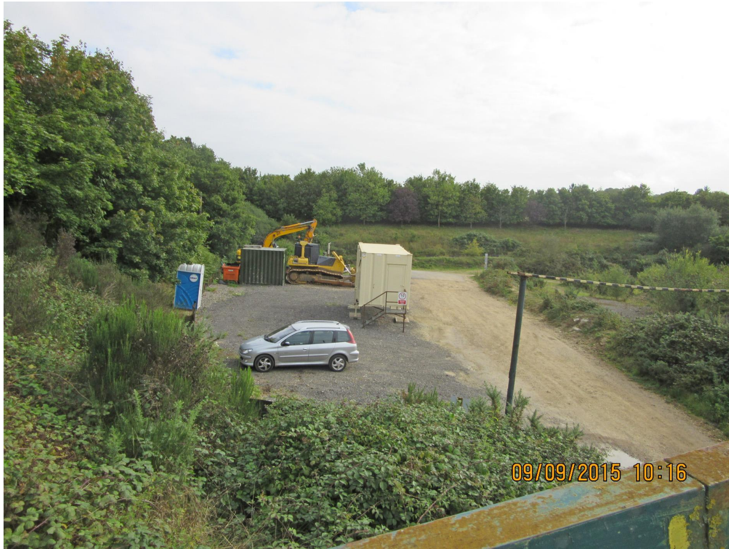
Figure 6 : View of staff welfare facilities on 9 September 2015, facing northeast
