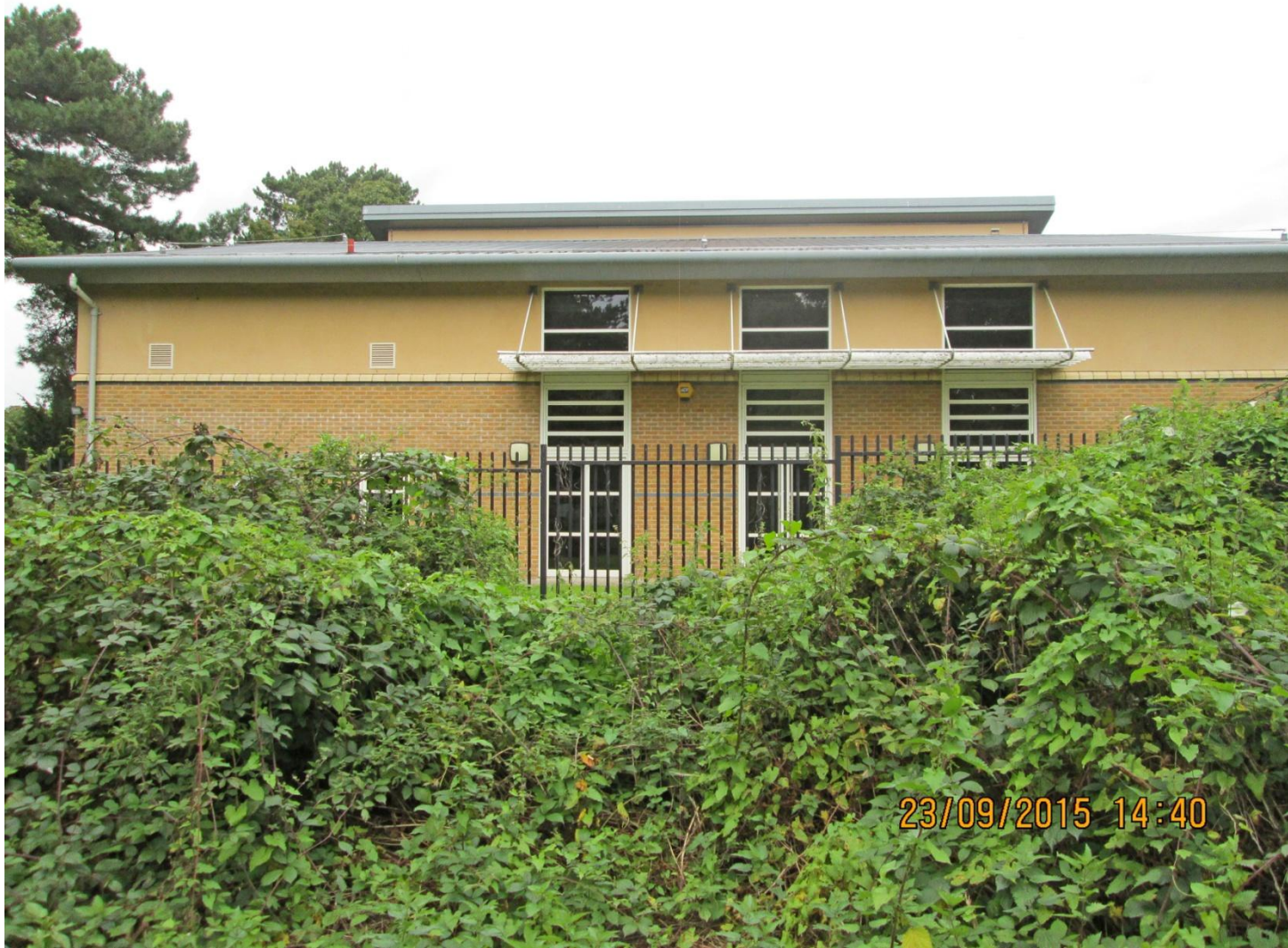
Figure 5 : Grammar school music block, viewed from proposed site compound / construction access
